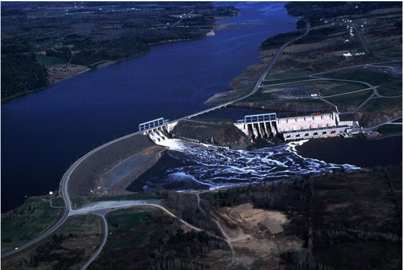
Mactaquac Hydro Electric Dam
